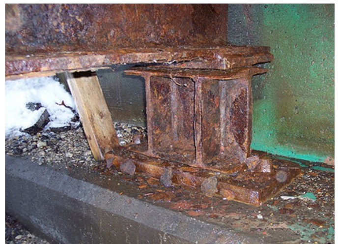
Fig. 1 Corrosion Affected Elements of a Bridge (Source: www.flickr.com [Tag: ascerportcard])
