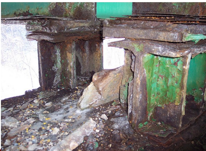
Fig. 1 Corrosion Affected Elements of a Bridge (Source: www.flickr.com [Tag: ascerportcard])
