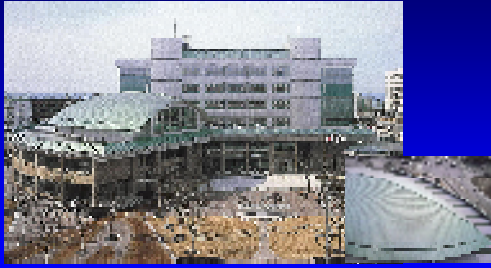
Uchinada Town Office/Ishikawa Prefecture, Japan - 1998 1,700 sq. m Roll dull & green color development 0.4 mm stepped roofing, titanium Gr. 1 sheet
