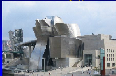
Guggenheim Museum, Bilbao, Spain Clad in polished titanium Grade 1 sheet Architect - Frank Gehry
