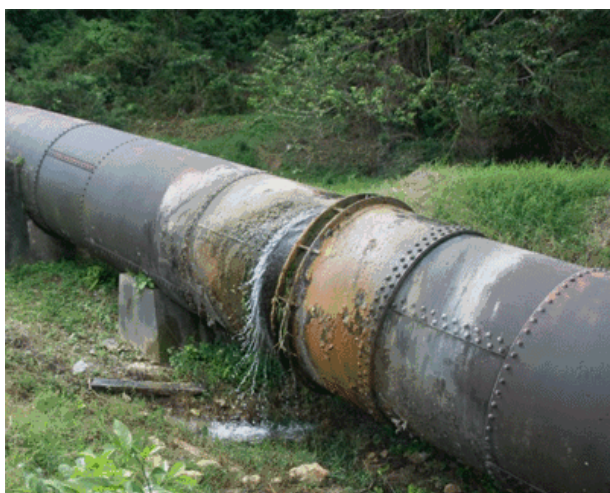
Figure 1: The aftermath of microorganisms accelerating pipeline corrosion.
